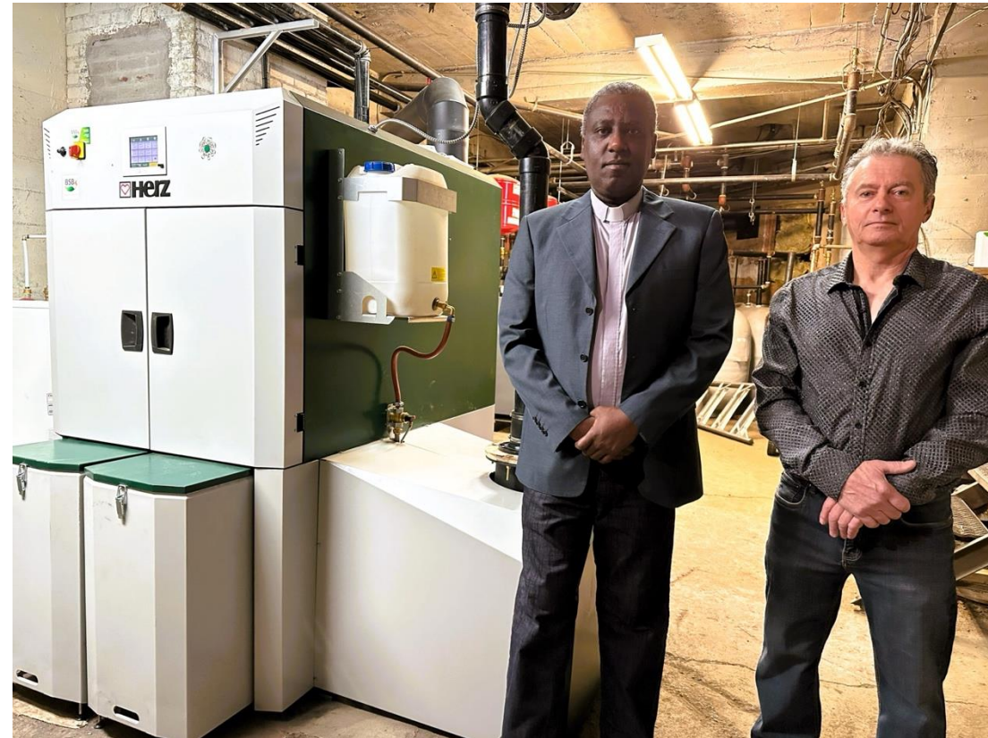
150kw boiler with 20 tonne silo and 2000 litre buffer tank
