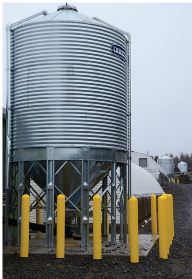
Three wood pellet silos were installed at the Kingsclear Provincial Tree Nursery last year, providing fuel for a trio of wood pellet boilers installed at the New Brunswick greenhouse as part of a retrofit. The boilers replace aging oil-fired boiler systems. Photo: Mark Rickard
