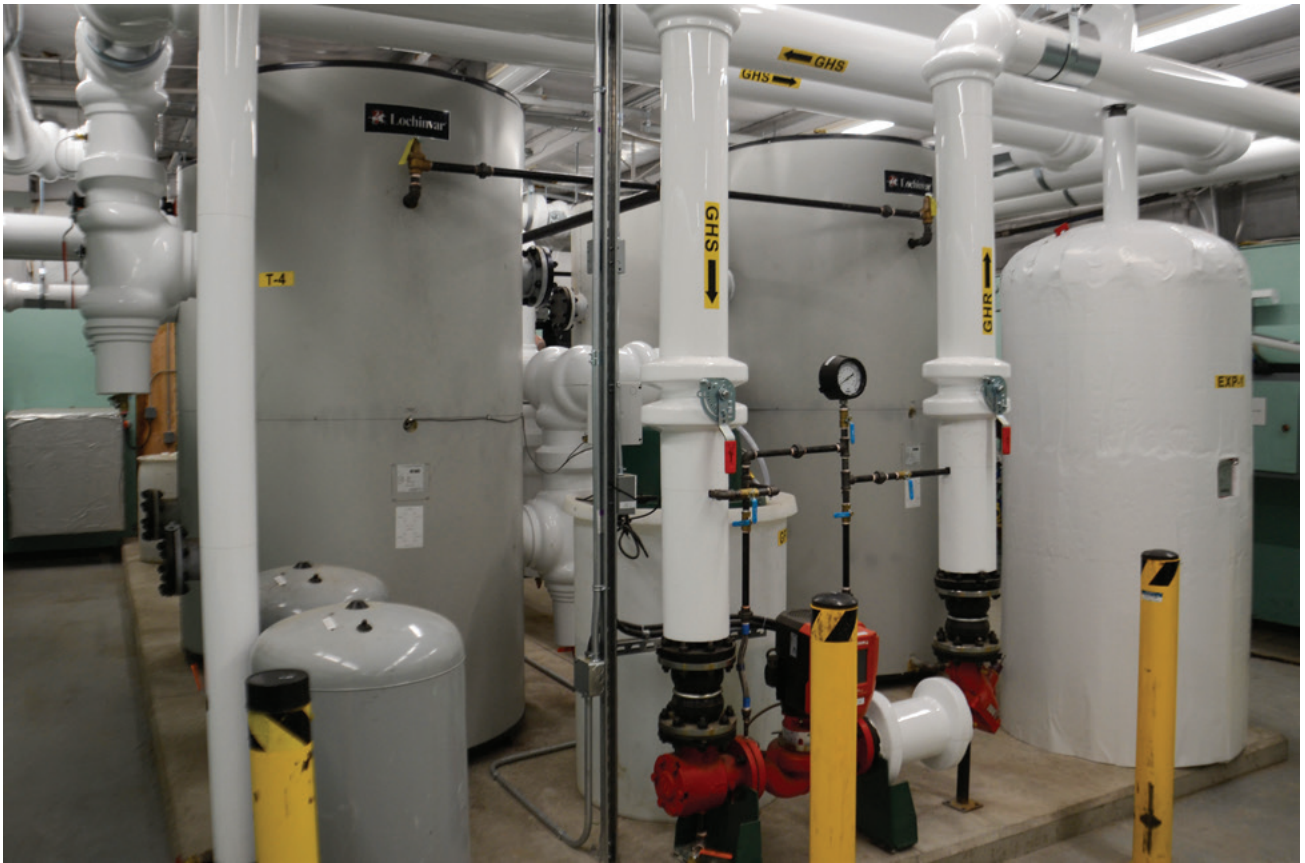
An extensive buffer tank system installed at the Nursery helps ensure tree seedlings can thrive despite a harsh New Brunswick winter. Three Herz Firematic 350 wood pellet boiler systems were installed at the facility as part of a retrofit. Photo: Mark Rickard
