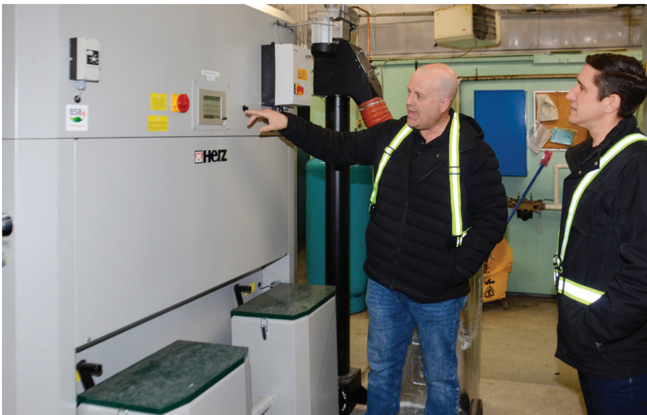
Jonathan Levesque, Biomass Solutions Biomasse (BSB) General Manager, explains some features of the Herz 350 Firematic wood pellet boiler system to Martin Noël, right, the Kingsclear Provincial Tree Nursery Manager. The provincial facility replaced three aging oil-fired systems with pellet boilers. Photo: Mark Rickard
