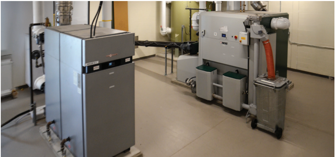
Hanwell Park Academy's boiler room was designed to use wood pellets. Photo: Mark Rickard
