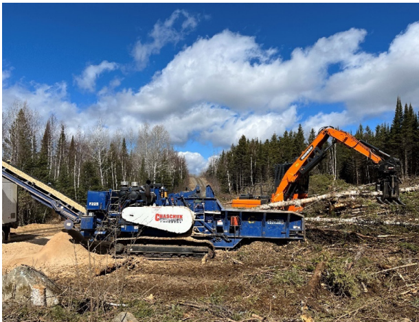
Figure 2 – Peterson 4710B Grinder on site
