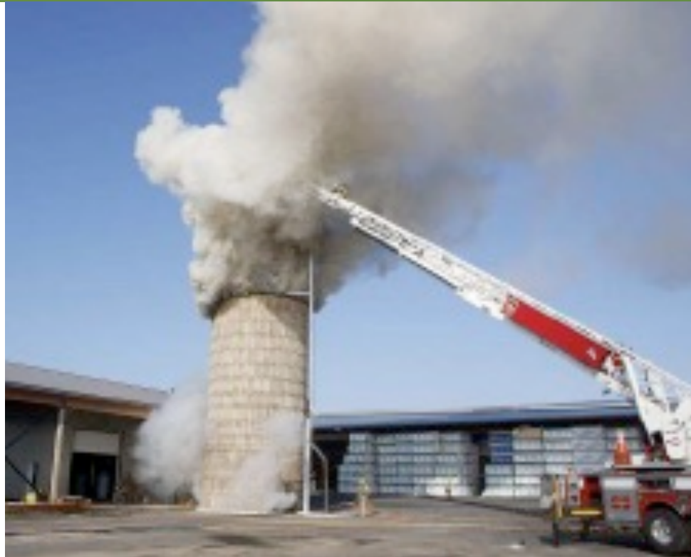
Fire in a silo containing wood chips; Lancaster, PA, December 2015; Lancaster Online.
