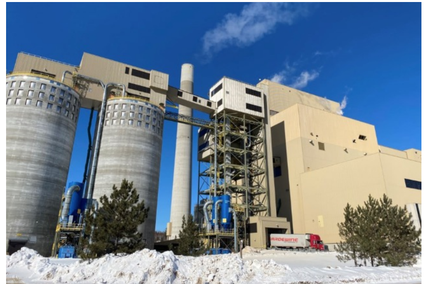
Atikokan Generating Station Photo: Ontario Power Generation
