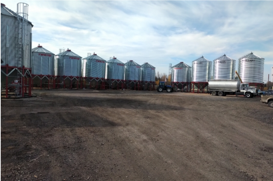
Figure 5: Pellet redistribution facility and pellet delivery truck, Norman Wells, NWT
