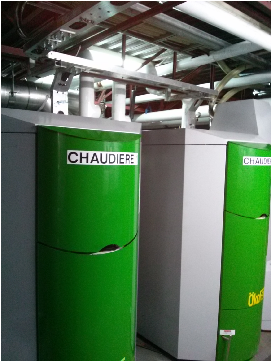
Figure 9: This is a two-boiler staged system heating a municipal building in the City of Clermont, Quebec.
