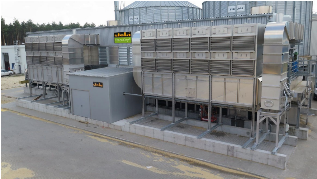
Figure D. 2. Stela's Indirect-heated Dryer with Hot Water Heat Exchanger Deck
