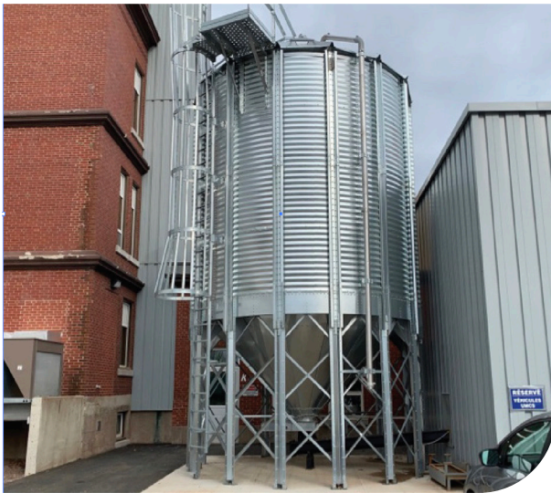
The farm-style silo holds approximately 30 tonnes of pellets and is refilled every 20 days in the depth of winter.
